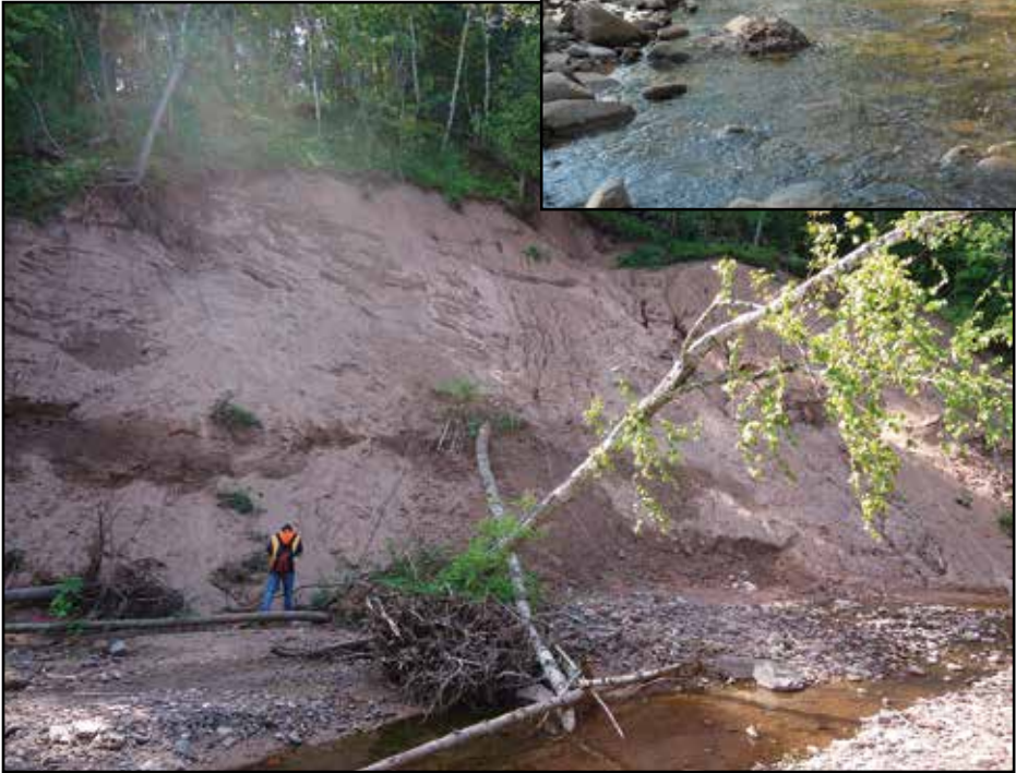
Left: Initial field survey in August, 2013. This slope failure is representative of others within the project boundary. Above: Same slope 1 year later; toe is stabilized with rootwads, live stakes, wattles, and native grass.
