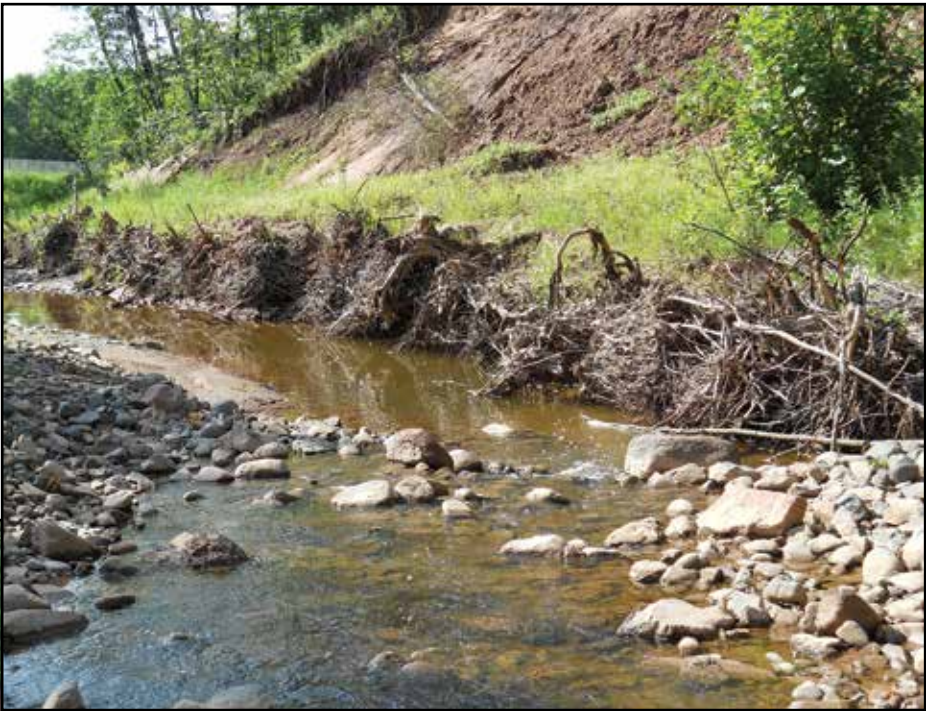
Left: Initial field survey in August, 2013. This slope failure is representative of others within the project boundary. Above: Same slope 1 year later; toe is stabilized with rootwads, live stakes, wattles, and native grass.
