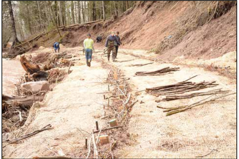
Above: Spring 2014 installation of live stakes. Below: South side of the debris catcher. The water in the photo is the original Mission Creek flow path. Woody debris bound up on the other side and caused the creek to carve a new flow path around the debris catcher.
