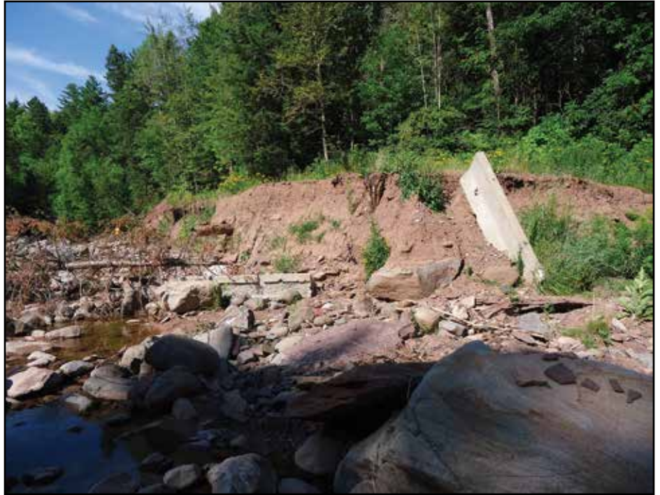
Above: This site is located at the upstream end of the project boundary. Note the concrete barriers embedded in the bank and channel bottom. Below: A bank that was stabilized by recreating a 3:1 slope and planting live stakes and native grass.
