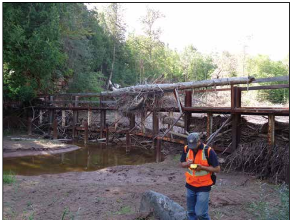
Above: Spring 2014 installation of live stakes. Below: South side of the debris catcher. The water in the photo is the original Mission Creek flow path. Woody debris bound up on the other side and caused the creek to carve a new flow path around the debris catcher.
