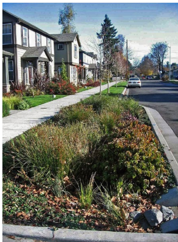
Green infrastructure elements require less area than traditional “gray” treatment structures and may be easier to insert in urban environments.
