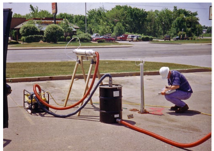
LimnoTech performs slug testing to measure local hydraulic conductivity, a necessary parameter for estimating the fate and transport of contaminants in groundwater
